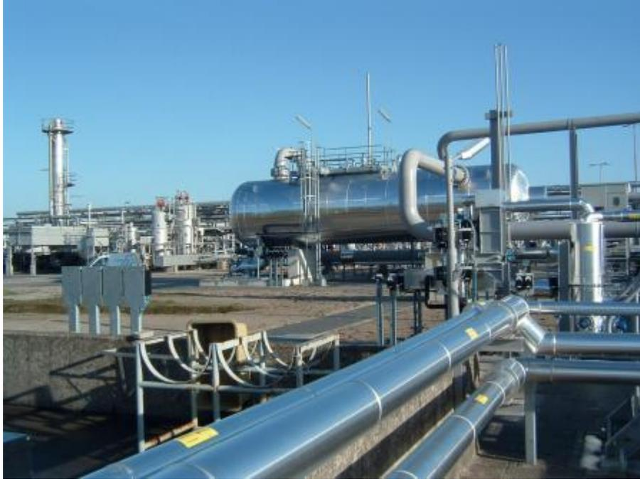
Pipeline specifications require removal of harmful acid gases carbon dioxide (CO<sub>2</sub>) and hydrogen sulfide (H<sub>2</sub>S) from the pipeline. H<sub>2</sub>S is highly toxic and corrosive to carbon steel. Carbon dioxide is also corrosive, reducing the BTU (British Thermal Unit) value of the gas. The natural gas desulfurization process can remove these acid gases, making natural a marketable product and suitable for transportation.
