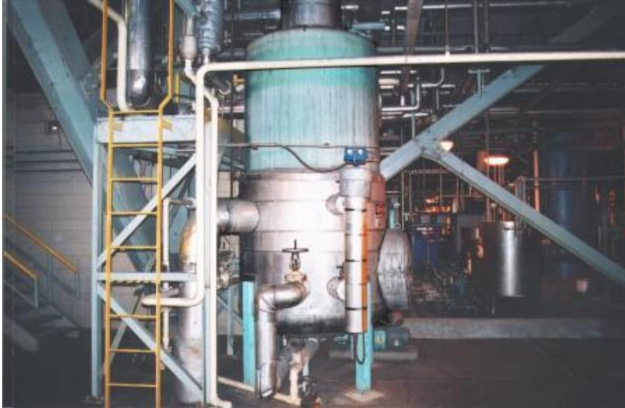
The concentration of undesirable solid particles in boiler water can be reduced by means of a continuous cleaning or draining system. The blowdown tank receives continuous discharge from the boiler drum and the discharge from the vapor generator at various temperatures and pressures. The waste tank can also be used as an automatic drainage system for the vapor generator when the generator is being drained for maintenance.
