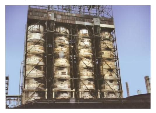
Coking is the ultimate means to transform the heaviest product of atmospheric and vacuum distillation. The feed is heated and cracked into light gas, gasoline mixture, distillate and diesel. The level applications for delayed and continuous (contact or fluid) coking include fractionator, light diesel stripper, vapor, condensate, discharge and sedimentation drums, and exhaust separation tanks.
