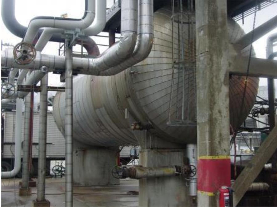
In the first stage of gravity separation, not all water is separated from crude oil. The water content of the separated crude oil may still be as high as 15%, and it is in the emulsifying state, so it is difficult to separate out again. The de-emulsification process is completed using chemical reagents and heating to eliminate the emulsifying state of oil and water in order to remove moisture before transporting crude oil.
