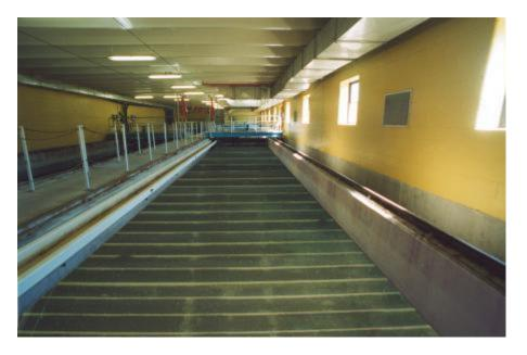
After the water treatment is purified, the pre-filtered water enters the filter bed from the inlet channel. When it passes through the medium of the filter bed-sand or deep filter type anthracite, cloth or surface filter type synthetic membrane, the fine suspended solids in the water are removed.
