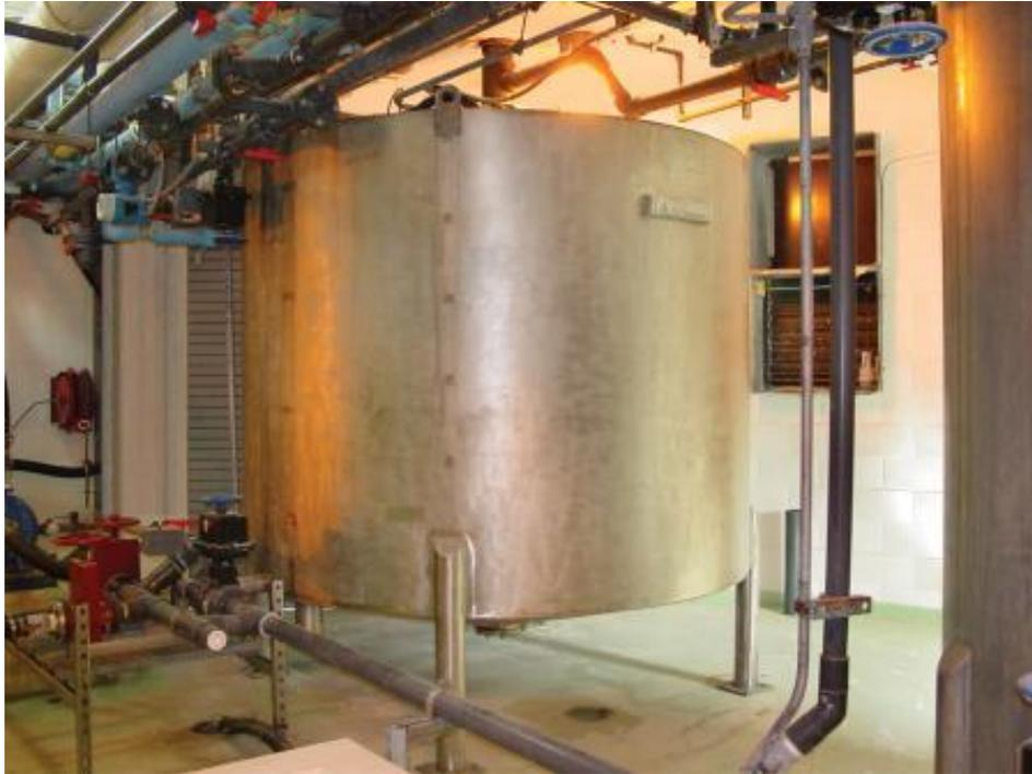
In terms of annual tonnage, lime consumption ranks first among water treatment chemicals. Lime is used for pH adjustment, phosphate removal, sludge and biosolid adjustment, etc., and is used in combination with other chemicals. Lime is initially mixed with water in a lime slaker to form a slurry called lime slurry. Then under strictly controlled conditions, the lime slurry is added to the raw water for formulation.
