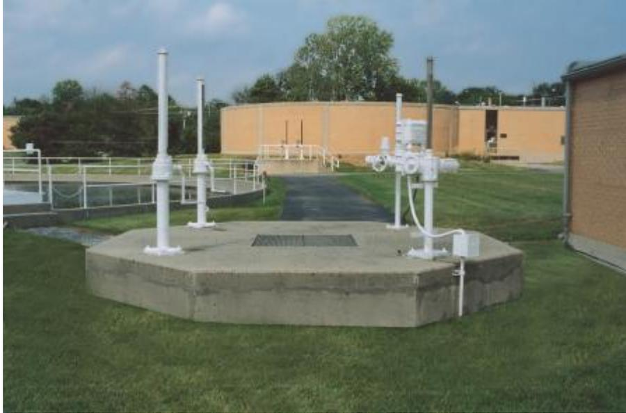
Wastewater treatment facilities have a large number of primary sedimentation tanks, usually using a concrete tank, which has compartments and doors, called a split box or distribution box, which divides the incoming water flow into multiple streams and transports them to the sedimentation tank. Similar devices can also be used to separate the mixed liquid flow between the secondary settling tanks.
