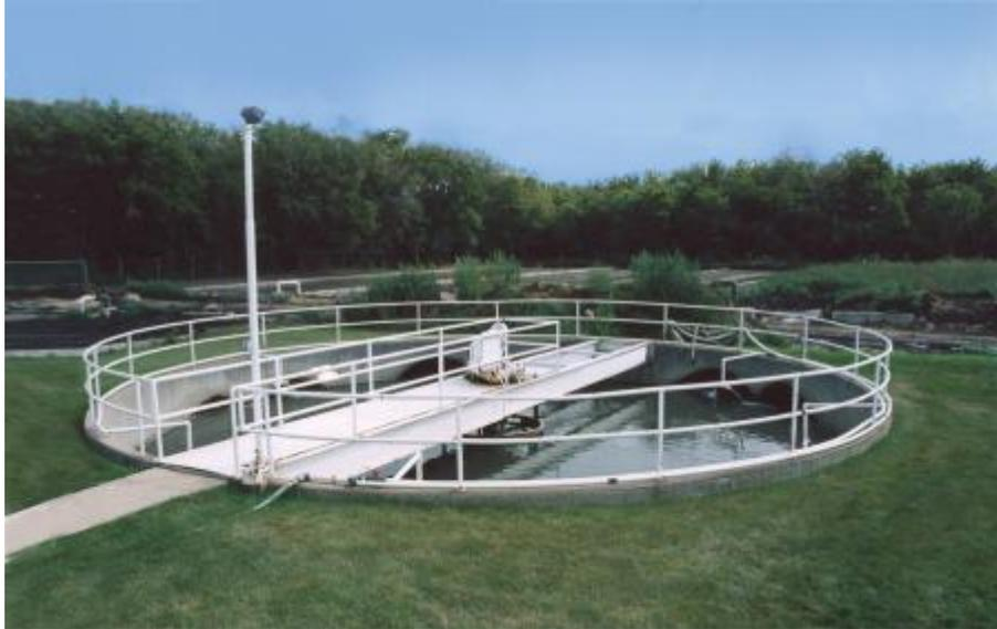
There is only one sedimentation tank in a small sewage treatment facility, and it is necessary to understand the surface level of the sedimentation tank. In larger sewage treatment plants, after the permeated water passes through the diverter box to reach many sedimentation tanks, there may not be enough space in the diverter box to accommodate the level gauge. In this case, the level monitoring of the sedimentation tank will help to obtain proper load balance.
