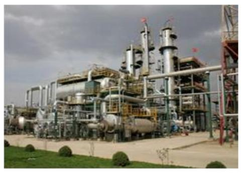
The unit is to recover sulfur from the acid gas containing hydrogen sulfide produced in the refining process with appropriate process methods. The advantage is to meet the requirements of product quality, reduce corrosion, and achieve long-term safe production of the unit with clean production, turning harm into profit, turning waste into treasure, reducing pollution, protecting the environment.
