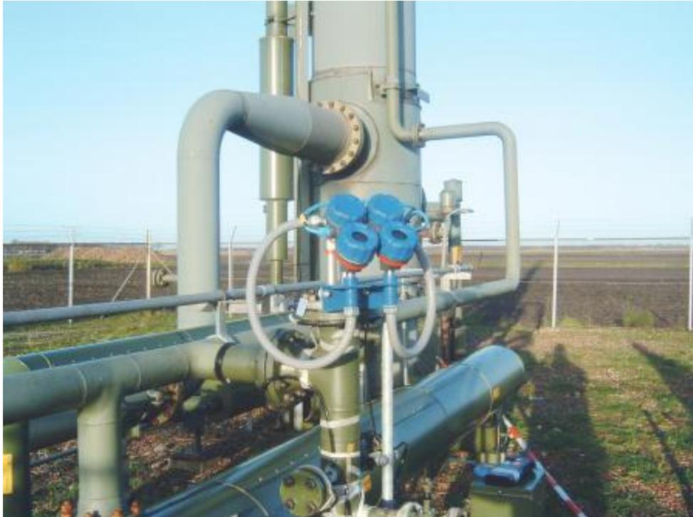
Where vapor-liquid separation is required, such as a separation drum, knockout tank, flash drum or compressor suction drum, will be integrated into the processing unit. The separation vessel receives a flash liquid mixture, and the liquid is subsequently separated by gravity, falling to the bottom from the top vapor outlet.
