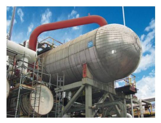
A column reboiler, or evaporator, is a heat exchanger that provides heat to the bottom of the distillation column. It boils the liquid at the bottom of the tower to produce vapor, which returns to the distillation column to drive the distillation separation process. A column reboiler may partially or completely evaporate the liquid collected at the bottom of the tower.
