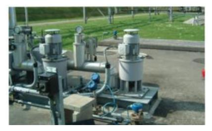
The scrubbers and filters of the air compressor station can capture waste liquid and harmful particles and transport the waste liquid to a storage tank. The waste liquid may be water condensate from natural gas or heavy hydrocarbons. Depending on the size of the remote air compressor station, the waste liquid is collected in one or several storage tanks. As the waste liquid tank is filled, a tank truck is usually arranged to empty the waste liquid tank regularly.
