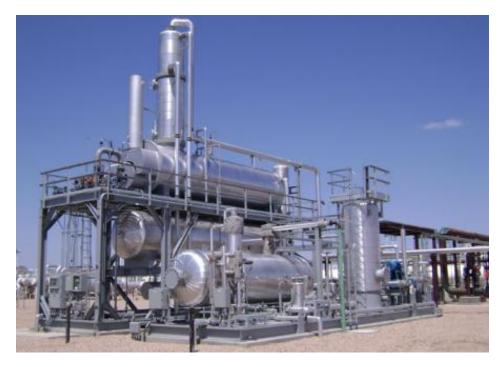
Natural gas needs to be dehydrated to remove hydrates to prevent these hydrates from crystallizing and blocking pipelines and obstructing the flow of gaseous hydrocarbon streams. Dehydration can also reduce corrosion, eliminate foam, and prevent problems downstream of the catalyst. Natural gas is dehydrated according to the customer's maximum allowable water content specification.
