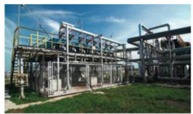
The sulfur recovery unit converts the hydrogen sulfide in the acid gas into elemental sulfur. Among these conversion processes, the Claus (two-stage desulfurization) method is by far the most famous elemental sulfur recovery method, while the traditional contact method and WSA method are the most commonly used technologies for sulfur recovery. The residual gas produced by the Claus process is often referred to as tail gas. The exhaust gas will be processed by the subsequent gas treatment device.
